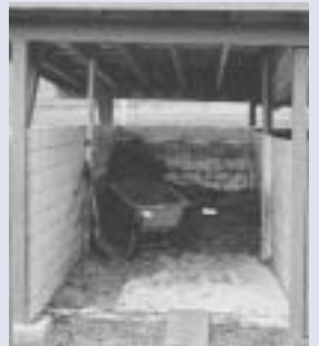
Store manure on an impermeable surface and under cover so that it doesn't leach into watercourses.
